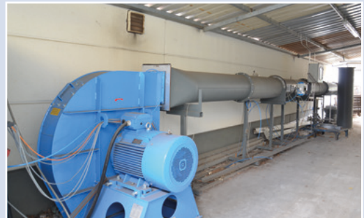
Test station at JASTA-ARMATUREN
